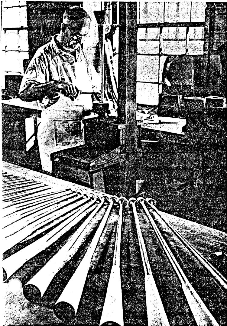
Reed Pipes Being Made in Pipe Shop
